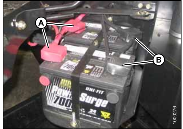
Figure 5.129: Battery Terminal Location
