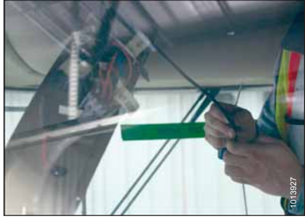
Figure 3.9: Fish Tape and Harness on Left Switch Panel Opening
