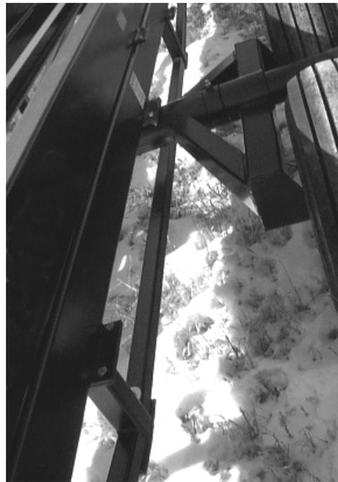
BOLT CENTER BRACE TO FRONT & REAR BRACE
